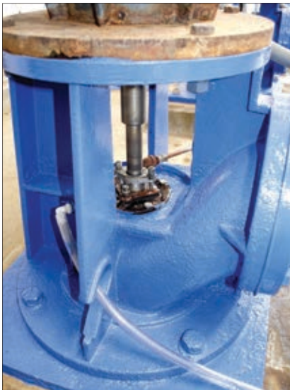
STAFF PHOTOS BY FINN HARTNETT A backwashing water pump uses additional water to cool itself down at Marion's water treatment plant.
