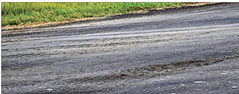
STAFF PHOTO BY PHYLLIS ZORN A blade patch surface on Remington Rd. shows grooves and bumps where the surface did not stick to the road’s undercoating.
